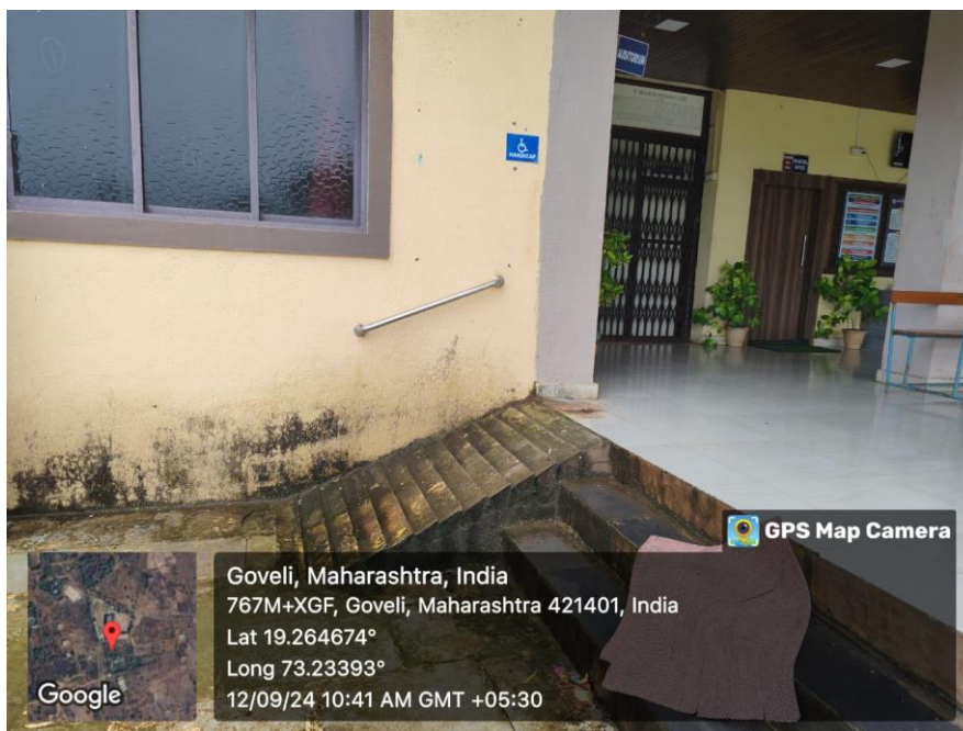
Ramps alongside steps for wheelchair access and guiding bars
